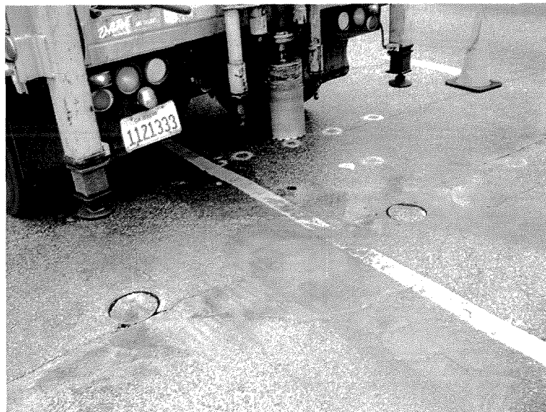
Figure 10: Existing pavement thickness determination Trench-in & Trench-out.
