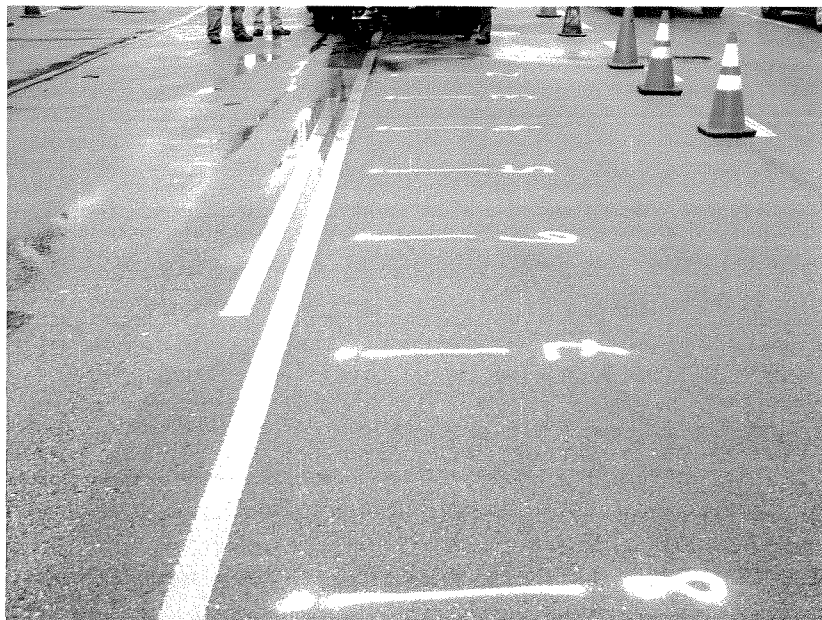
Figure 3: Shows FWD to be measured in a control area with consistent Asphalt thickness structure.
